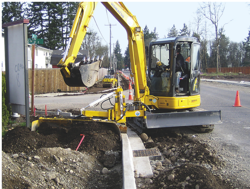
Hinged anchor at the corner of the backfill blade is supported by a strut spanning from the end of the blade to the rear of the track frame. Caster wheels follow the curb for reference.
